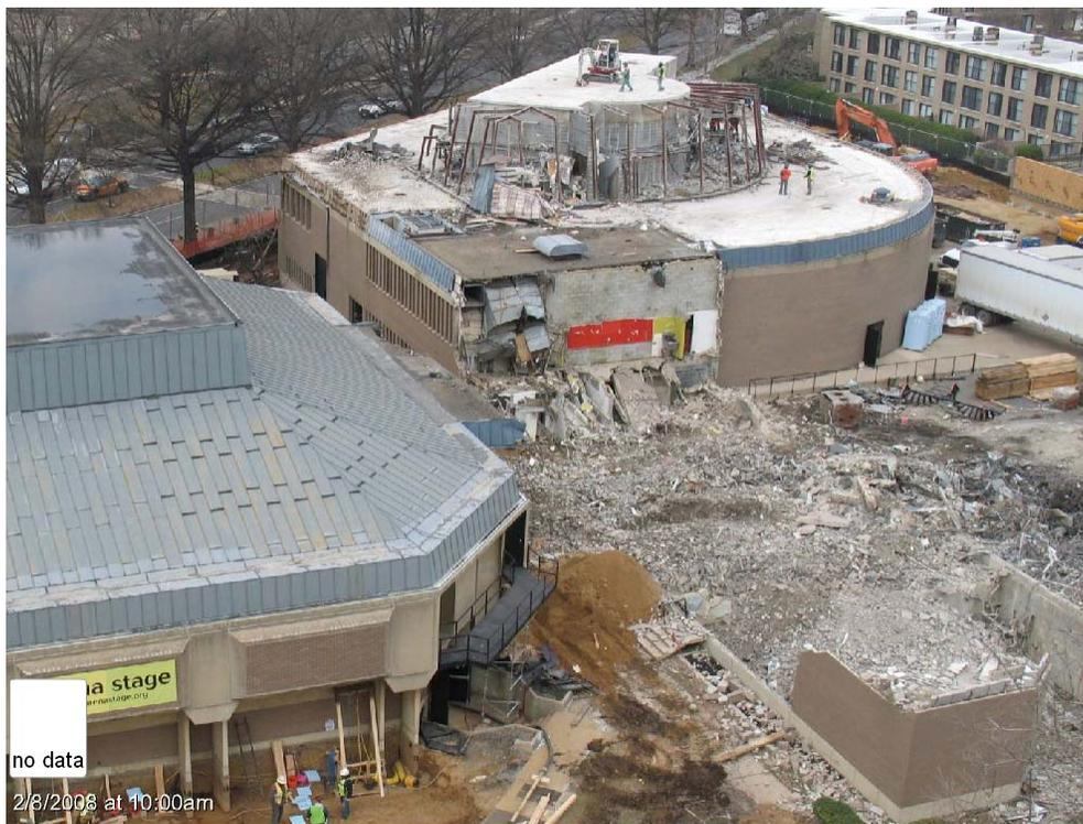
**Figure 1:** Arena Stage during selective demolition in February 2008
